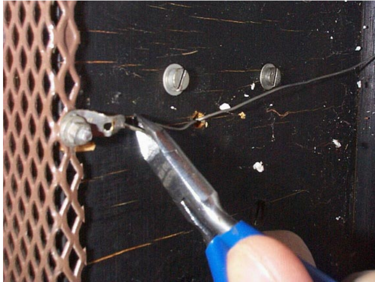
Figure 3.2: Cut Grille Grounding Wires
