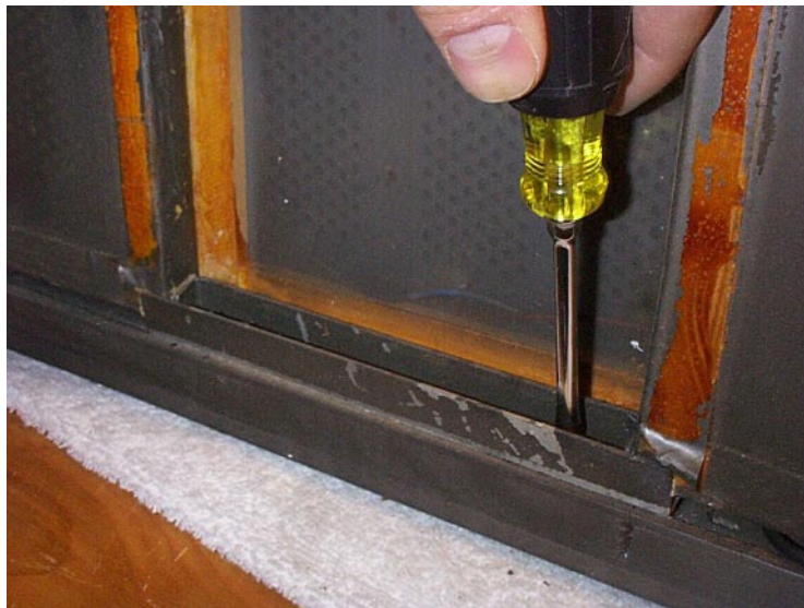
Figure 3.11: Removal of Panel Retaining Brackets
