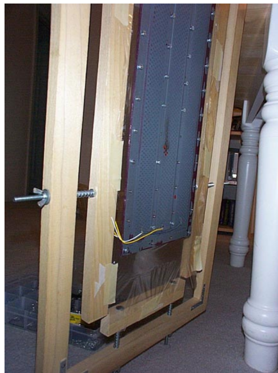
Figure 5.21: Bolting Treble Panel Together with 3/8'' 4 – 40 Bolt Assemblies
