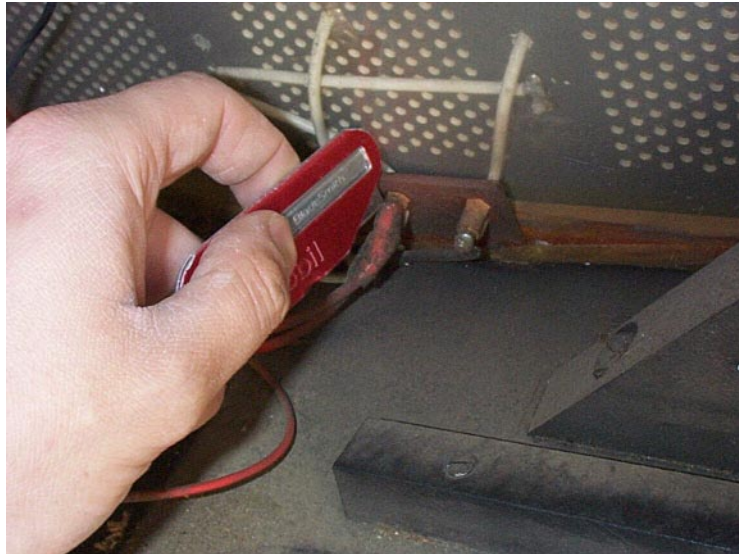
Figure 3.17: Cut Bias Wiring Insulation
