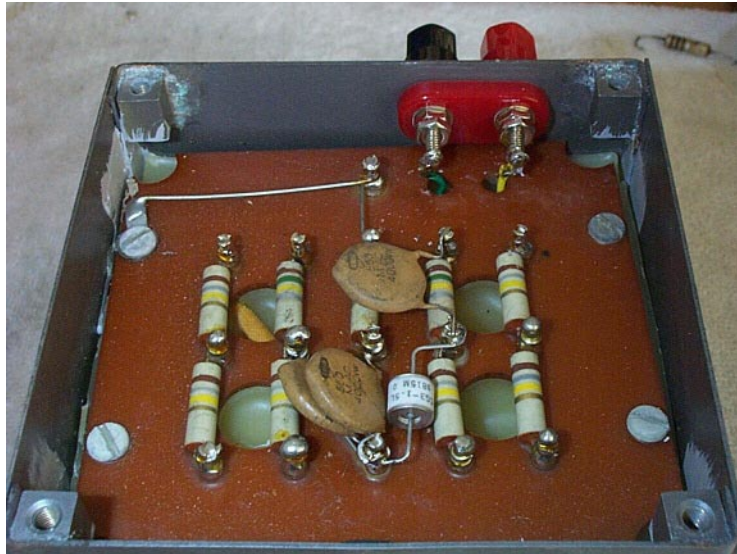
Figure 7.4: Finished Input Transformer (With Gas Discharge Tube)
