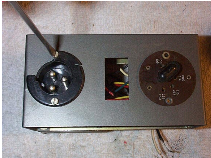
Figure 6.13: Unscrew Broken Bulgin Connector
