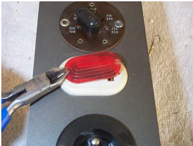
Figure 6.11: Carefully Removing Neon Bulb Cover Retaining Rivets
