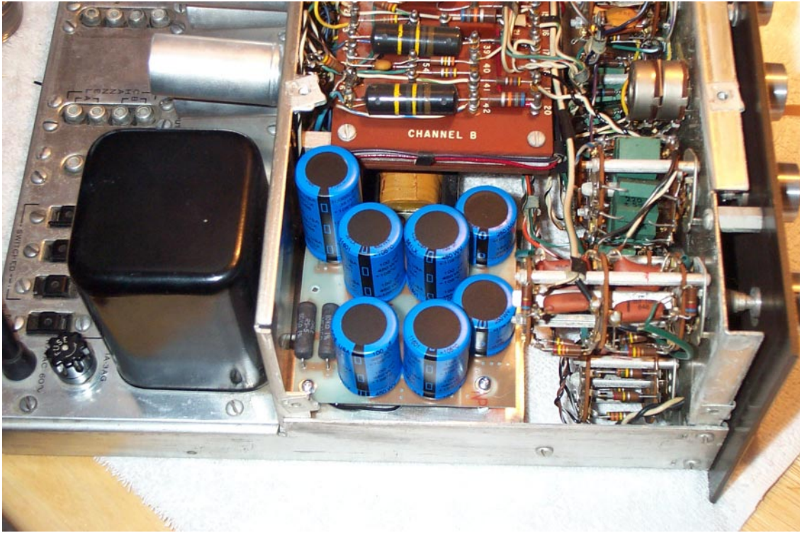
Capacitor Board Installed in Amplifier
