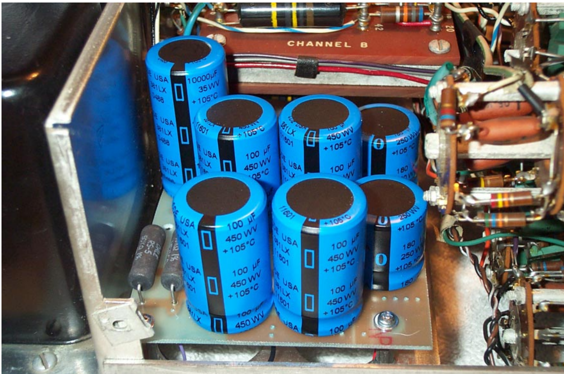
Capacitor Board Installed in Amplifier
